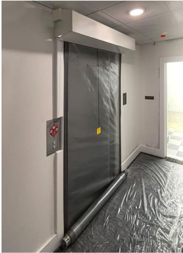
Hoistway Protection - Section 3006.2
